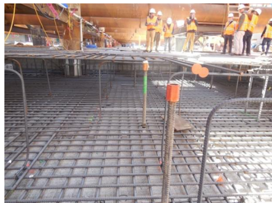
Reinforcement of bottom plate
