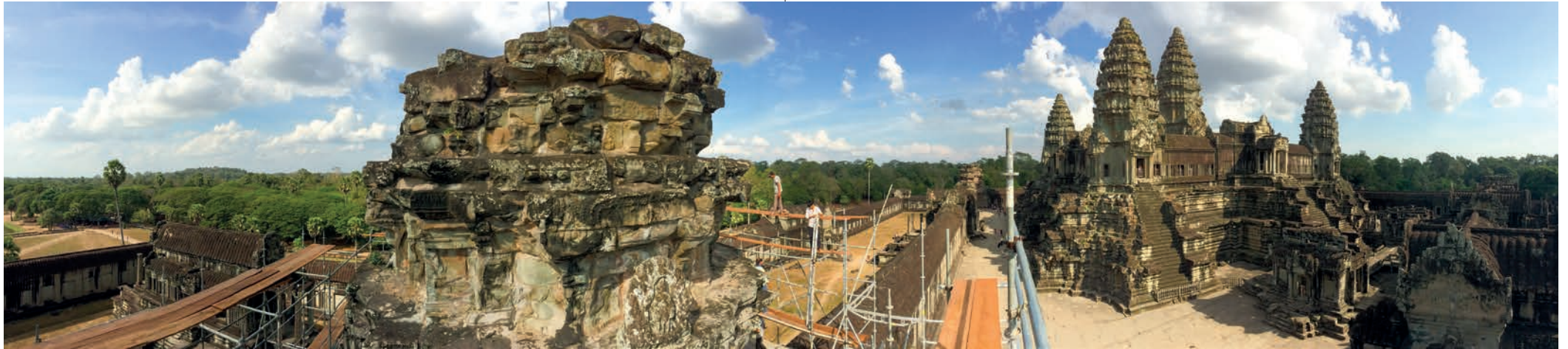
New GACP scaffolding at North West tower, 2nd level at Angkor Wat 2017
